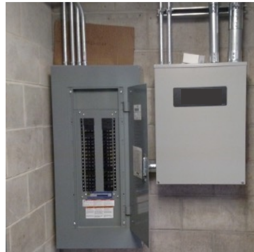
Example Transfer Switch
