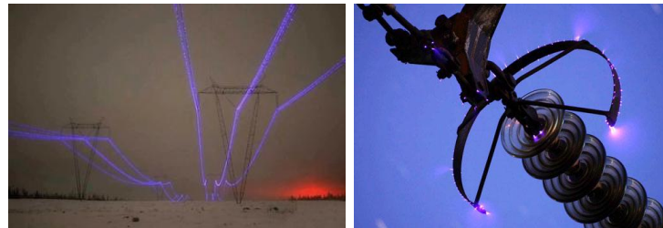
Corona effect shown as a visible glow (Image credit: https://electronicslovers.com/2018/07/corona-effect-can-influence-the-overhead-transmission-lines.html )
